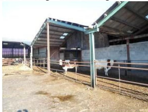
Farm building – Cattle housing
