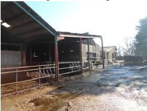
Farm building – Cattle housing
