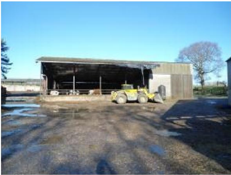
Farm building – Cattle housing
