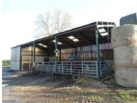
Farm building – Cattle housing
