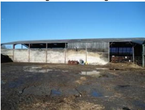
Farm building – Cattle housing
